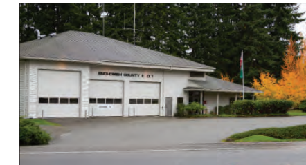
Station 13 / Silver Firs 13611 Puget Park Drive Everett WA 98208
