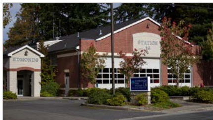
Station 16 / Edmonds Maplewood 8429 196th Street SW Edmonds WA 98026
